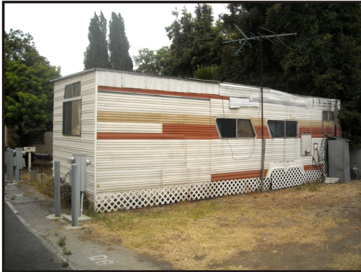
View of existing trailer homes.
