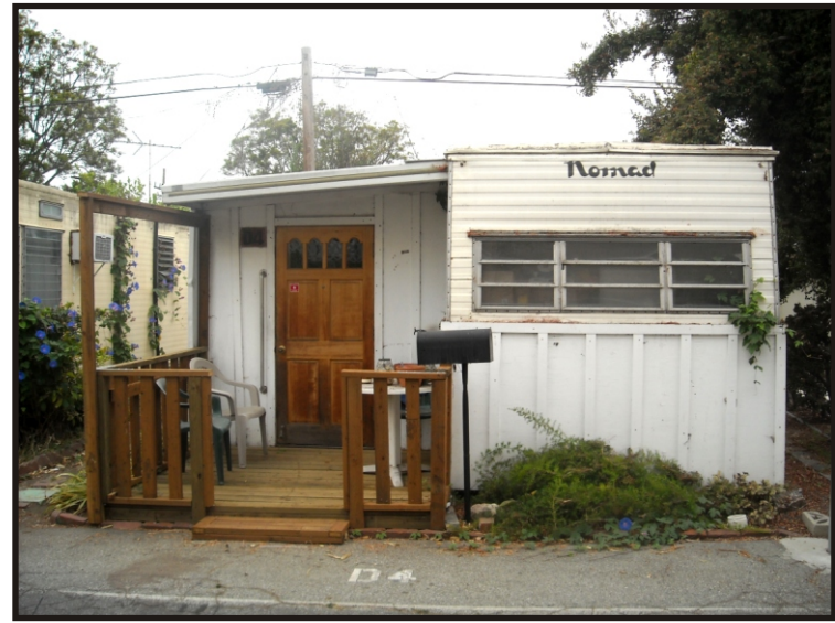
View of existing trailer homes.
