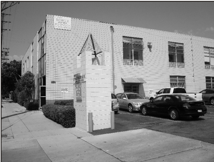
Looking east at adjacent building to the west.
