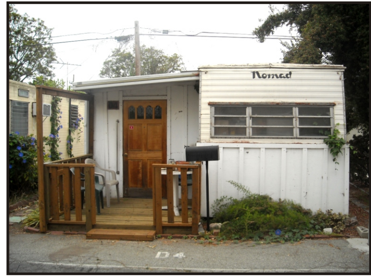
View of existing trailer homes.
