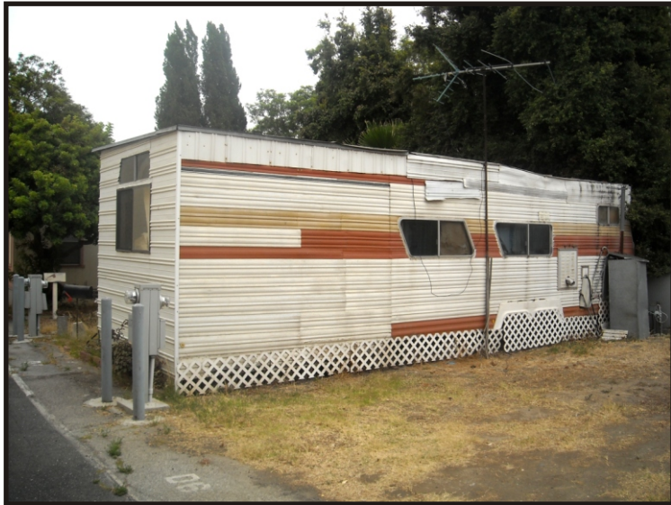
View of existing trailer homes.
